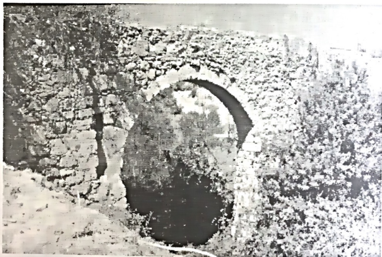
Figure 11 - Aqueduct at Zeytinlik (Templos), Girne.
