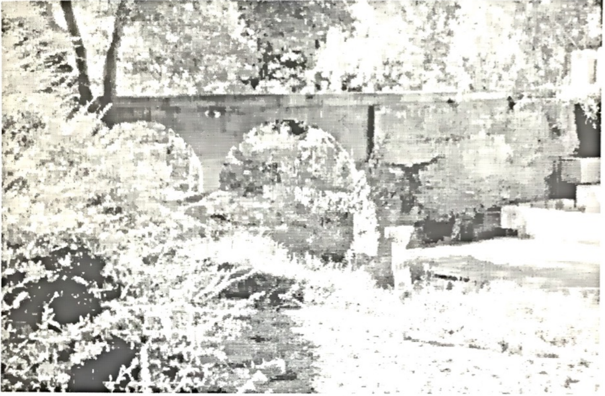
Figure 12 - Aqueduct at Alsancak (Ay Yiorgios), Girne.
