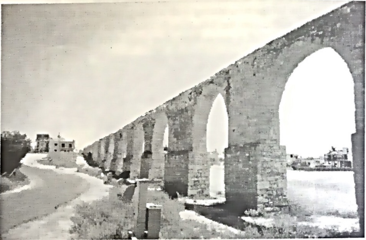
Figure 6 - Bekir Pasha Aqueduct. Larnaca.
