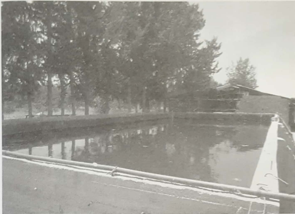
Figure 9. The water tank contains 1000 tons of water. It is fed by underground wells and it serves to irrigate the farm.
