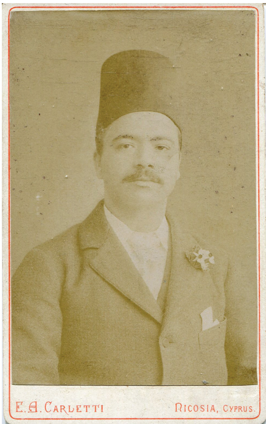
Figure 1: E.A. Carletti. Unidentified, 1880s. Courtesy of Balkanphila Ltd.
