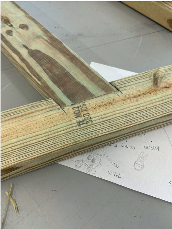
Figure 5 Let-in framing joint in pressure-treated wood.
